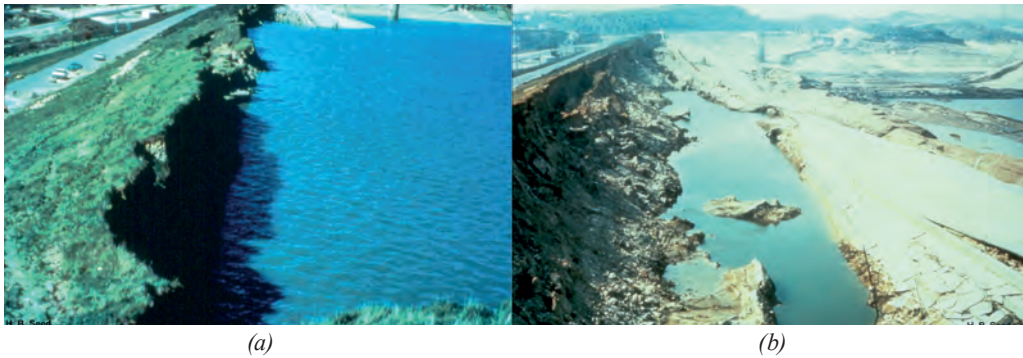
Figure 6. Lower San Fernando Dam, upstream face showing liquefaction slide due to earthquake (M 7.1) shaking, a) immediately following the earthquake; b) after the reservoir was drawn down [17]
