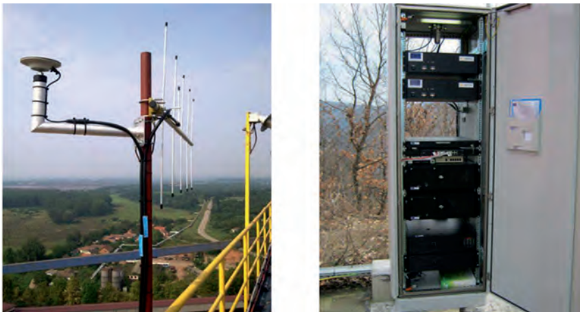
Figure 10. AIS base station, Serbia [30]
