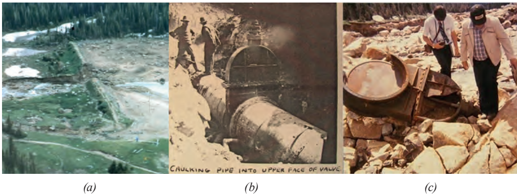
Figure 4. Lawn lake a) embankment after failure; b) gate valve improperly installed; c) recovered gate valve 70 m downstream [14]
