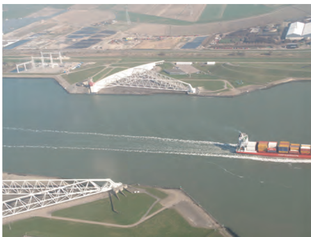
Figure 2. Maasdijk, tide gate at Rotterdam [7]
