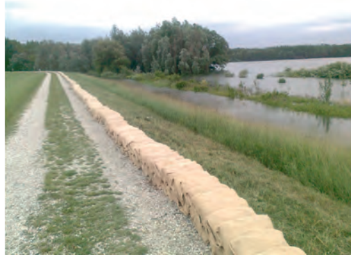
Figure 22. The correctly prepared protection line made of filled sandbags (photo archive of NYUDUVIZIG)
