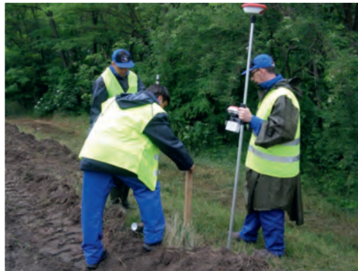
Figure 7. In case of heightening the levee, its height must also be marked (photo archive of NYUDUVIZIG)
