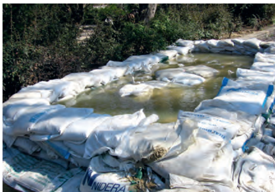
Figure 20. Counterpressure basin over a manhole, the overflow is not necessary in this case (Budapest Sewage Works Ltd.)
