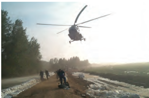
Figure 26–27. Placing sandbags by helicopter during the flood in 2013 in Győr (photo archive of NYUDUVIZIG)
