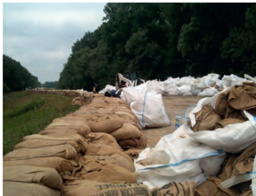
Figure 18. The most important material of flood protection is the sandbag (photo archive of NYUDUVIZIG)
