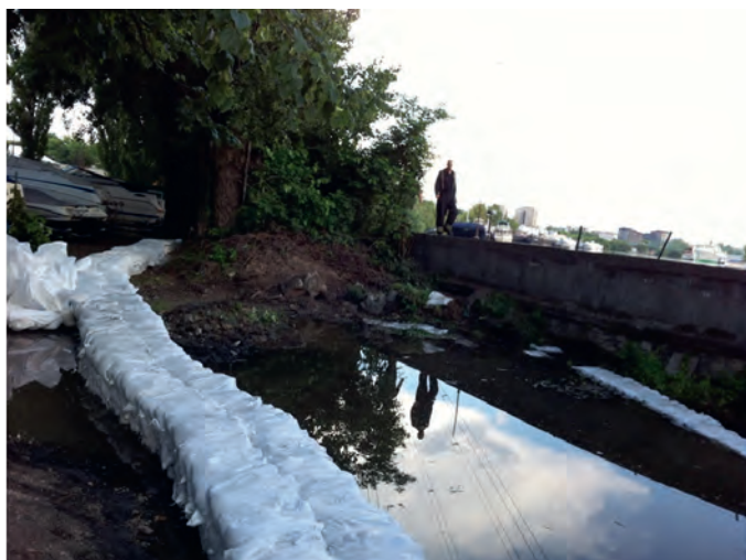
Figure 16. High flood protection wall, seepage control by counterpressure basin, Budapest, 2013 (Budapest Sewage Works Ltd.)
