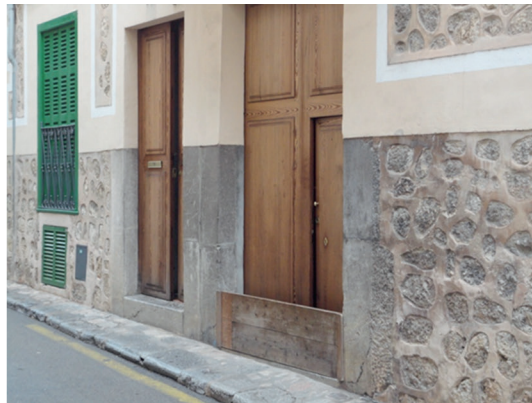
Figure 16. Elevated door sill and door flood barrier at Sóller in Mallorca (photo taken by the author)
