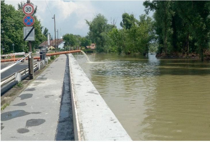
Figure 36. Excess water control in an unplanned place in 2013 (photo archive of NYUDUVIZIG)
