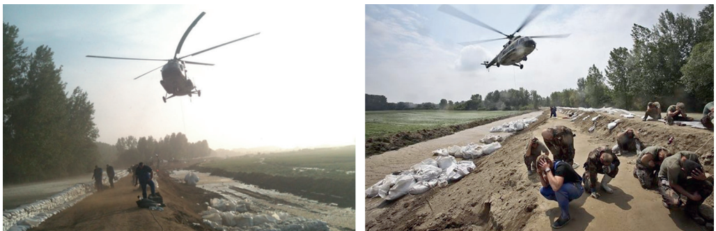
Figure 26–27. Placing sandbags by helicopter during the flood in 2013 in Győr (photo archive of NYUDUVIZIG)
