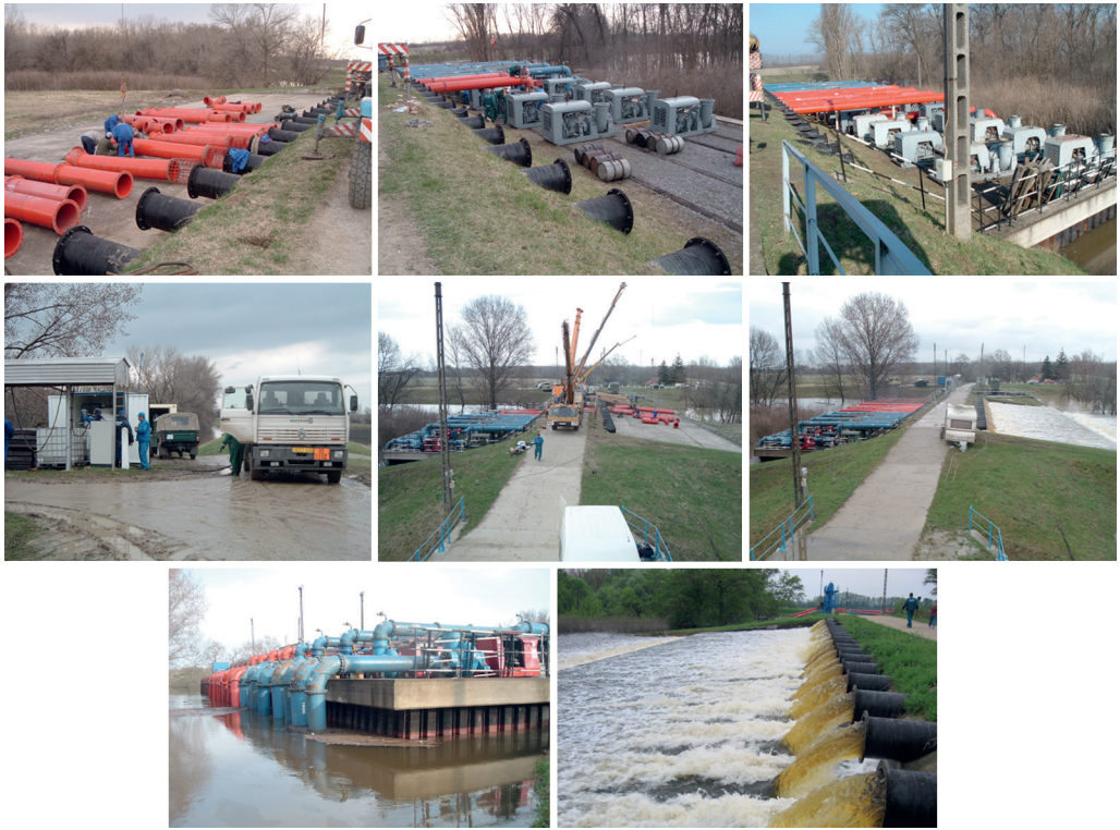
Figure 37. The temporary portable pump during the excess water control in the spring of 2013 (photo archives of TIVIZIG, KÖVIZIG and KÖTIVIZIG)
