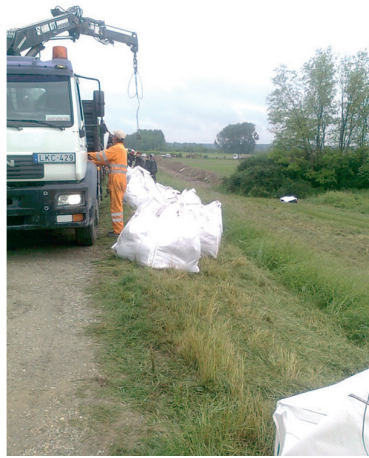
Figure 23. Protective material transport on the dyke (photo archive of NYUDUVIZIG)
