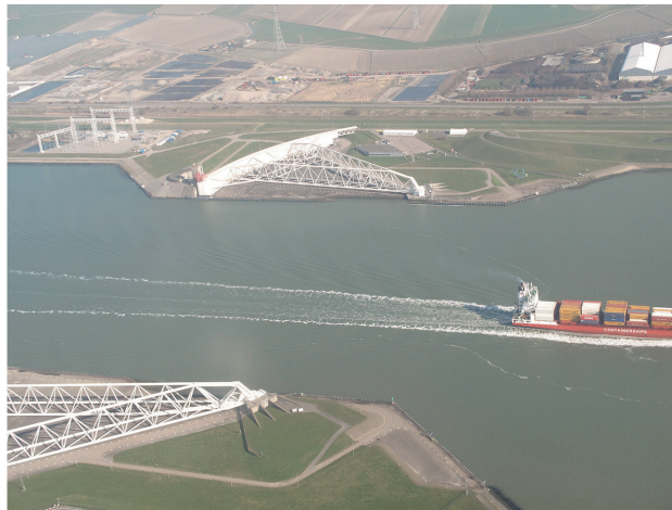
Figure 2. Maasdijk, tide gate at Rotterdam [7]
