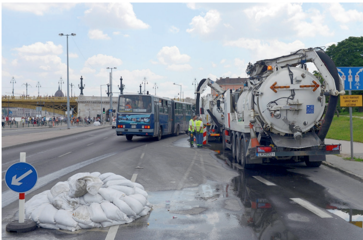
Figure 19. Weighting of manhole during the 2013 Budapest flood (Budapest Sewage Works Ltd.)
