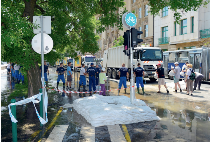
Figure 18. Weighting of underground railway by vehicles (buses and garbage collecting lorries) in a highest ever flood, 2013 Budapest (Budapest Sewage Works)
