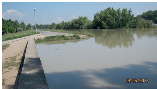
Figure 12. Earth dyke at the cross section change in Budapest, Pünkösdfürdő in the 2013 flood (Budapest Sewage Works Ltd.)
